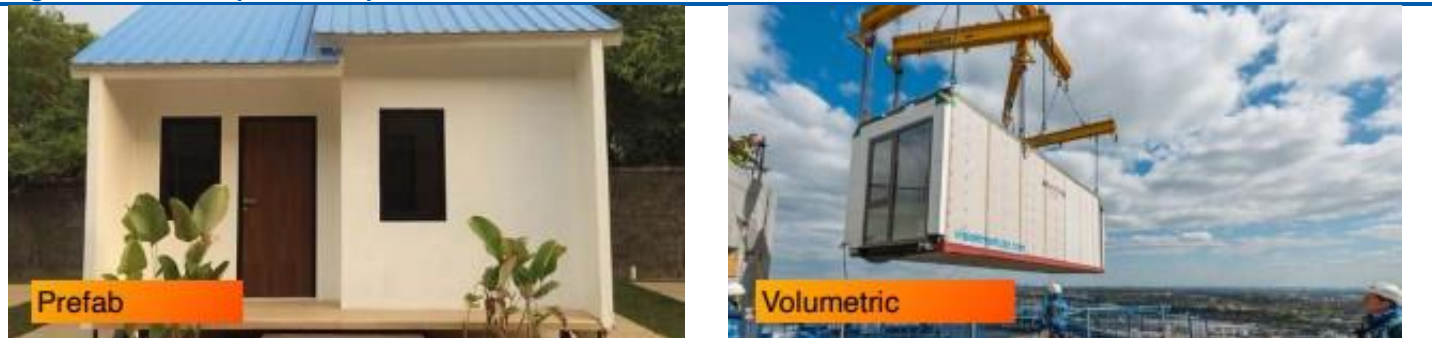
Figure 61: Modular products – prefab and volumetric
