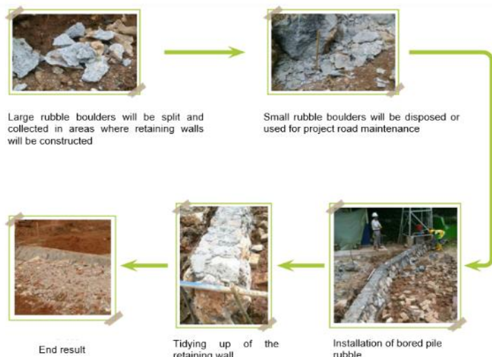
Figure 58: Process of using recycled concrete pile
